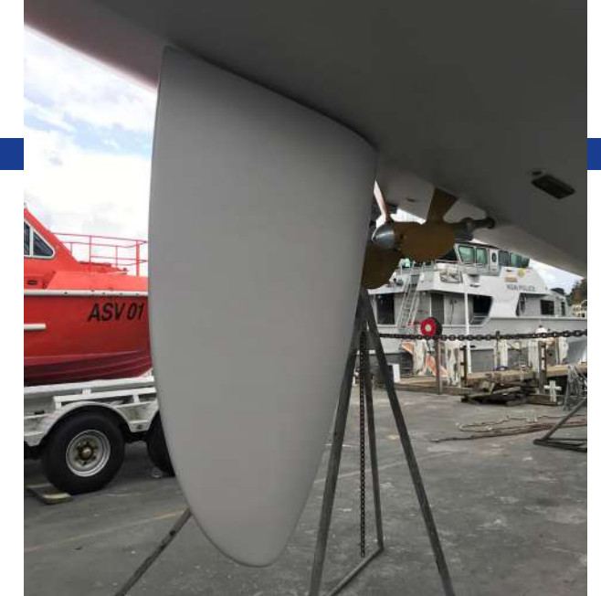
Rudder removal is required to inspect stock.
