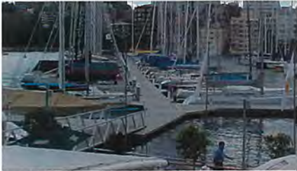
Arm A of the CYCA – part of a world-class facility
