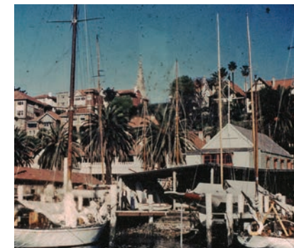
The front of the Clubhouse in 1956 before the many additions to the marina and Club building
